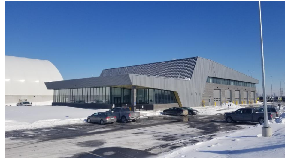
Rebuild of Steeles Patrol Yard
